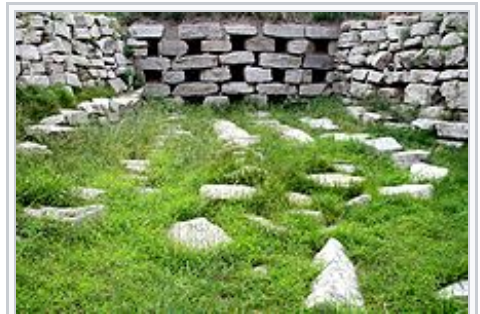
Remains of Ancient Linzi city sewer □ passing underneath the former city wall of the Qi kingdom.
